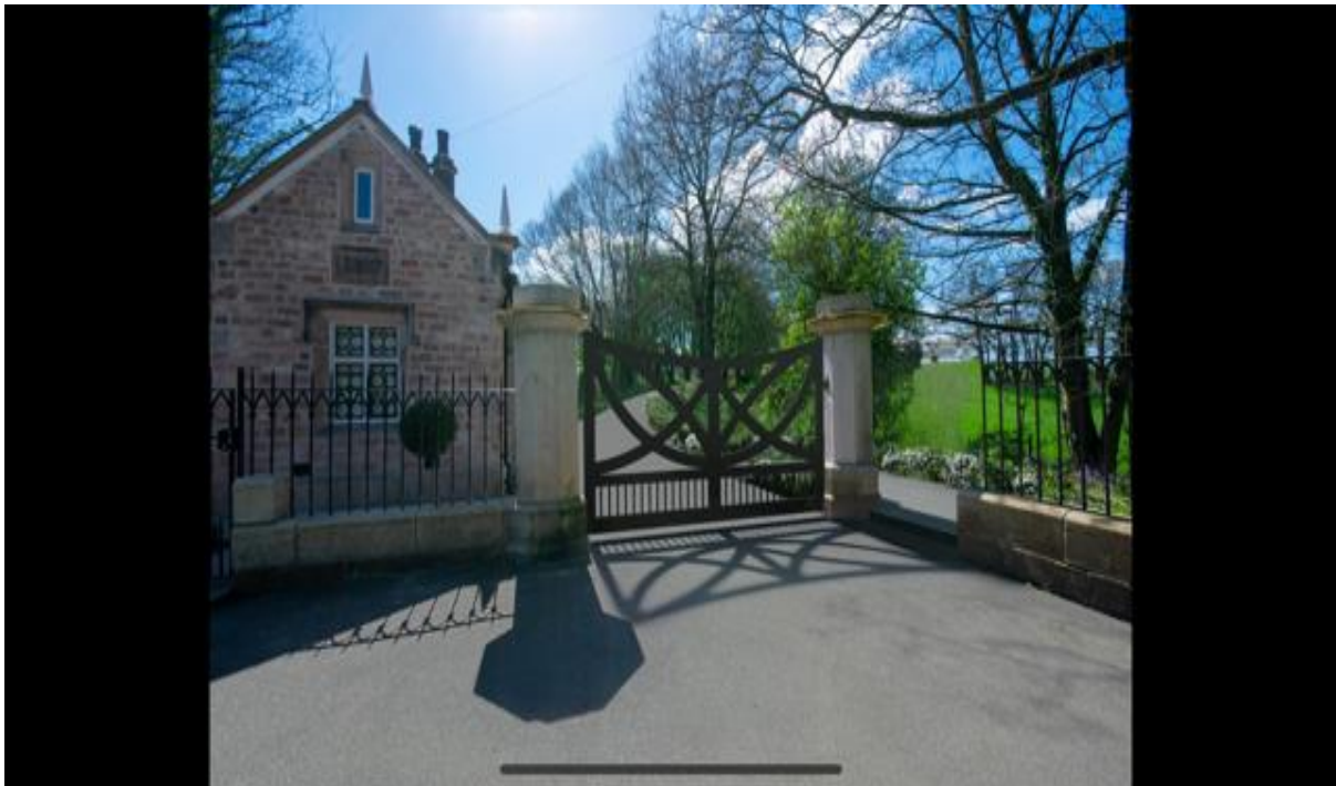
Image Showing the New Gates Renovated Walls/Fences and the New Pedestrian Access.
